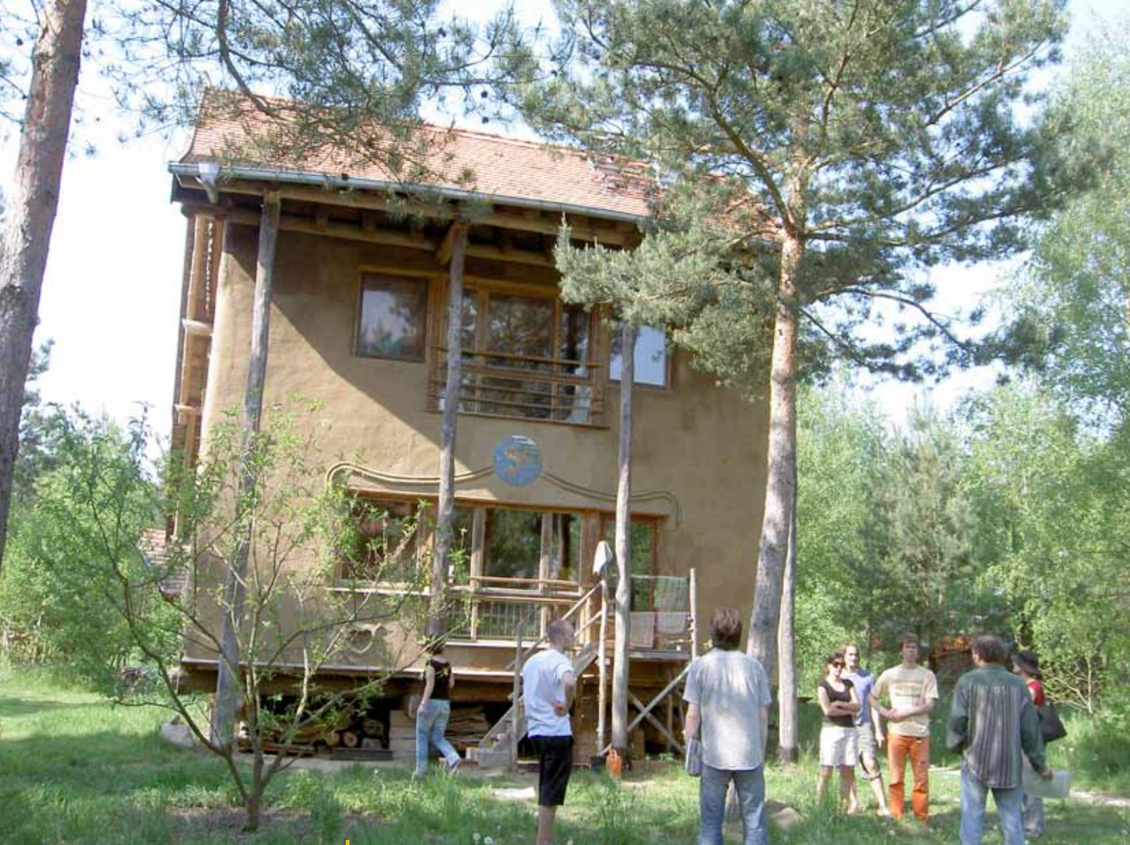
A 'handmade' strawbale house in the Ecovillage of 'Sieben Linden'.
